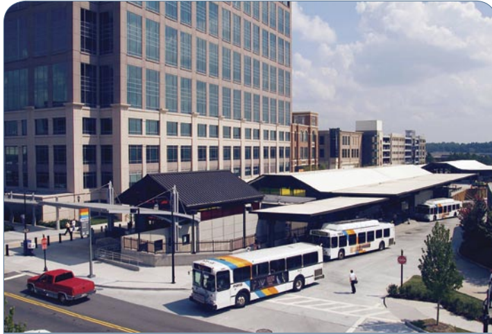
The Lindbergh MARTA station has become the focal point of a transit-oriented development that Peggy Whitaker fought to improve.
